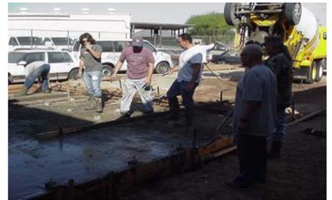
A Building Construction class poured concrete as part of a lab project that will be used in the Industrial Technology Division. Students got hands-on experience in learning methods of pouring and finishing concrete.
